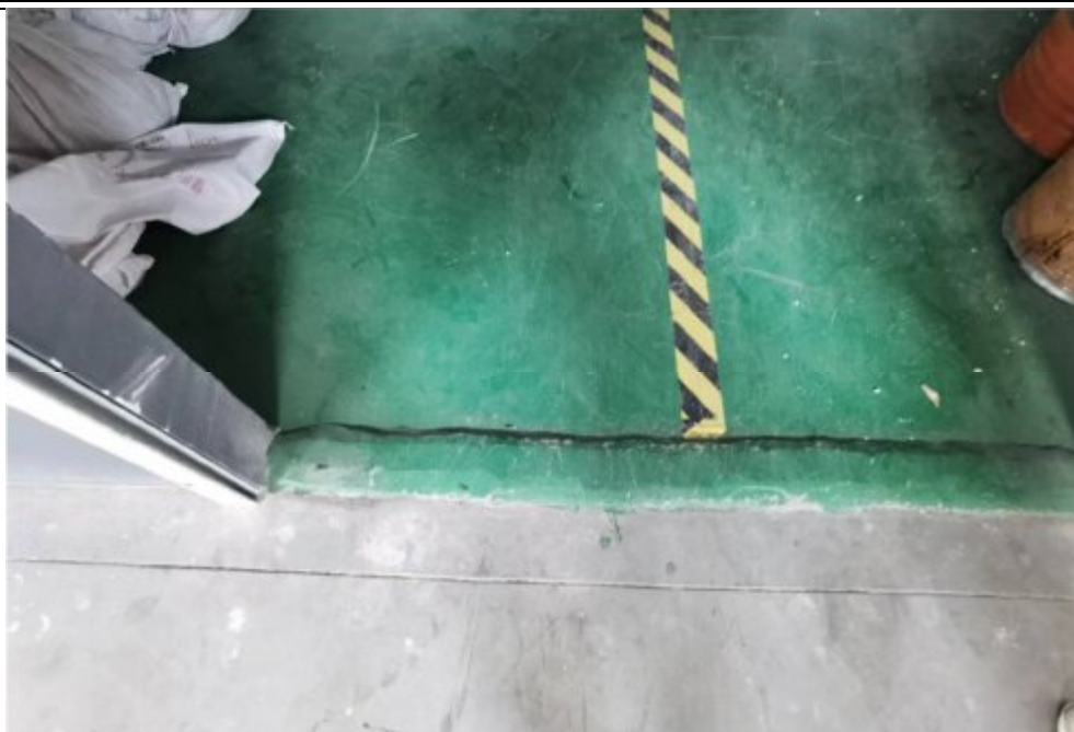
危废仓库门口斜坡
